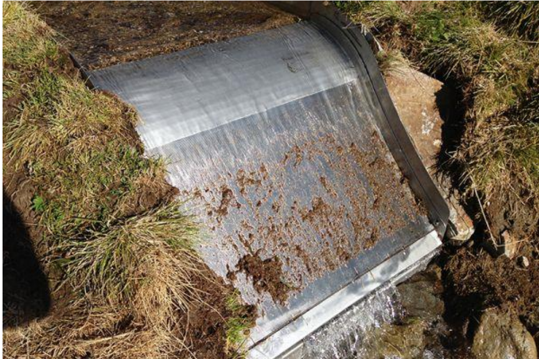
Figure 9. Sediment movement on Coanda intake (Source: https://www.wild-metal.com/sites/default/files/styles/contentbilder/public/referenzbilder/prischeralm_wildmetal_stahlwasserbau.jpg?itok=t6TEy0qN )
