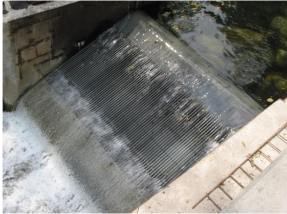
Figure 5. Tyrolean intake (Source: https://www.braun-tech.com/upload/filecache/Basochhu_1_4eb43d92e9a2bc8ff3922a78b0c6a30a.jpg )
