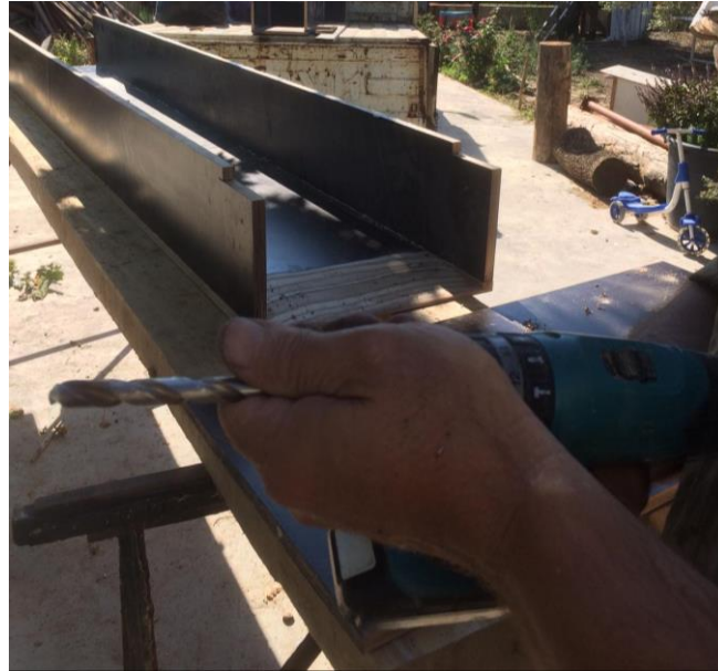
Figure 43. Photo of the main flume taken during its construction process
