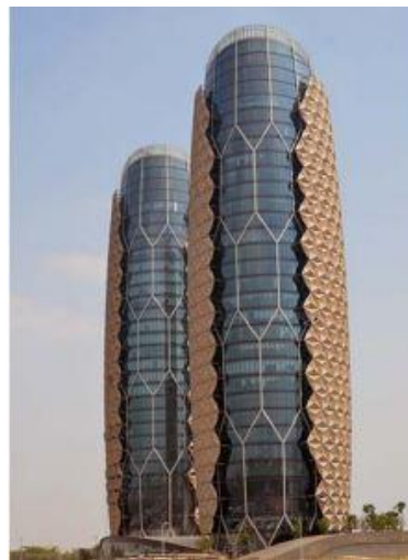
Figure 2.6. Al- Bahr Tower with dynamic Shading Systems (Source: Attia, 2018)
