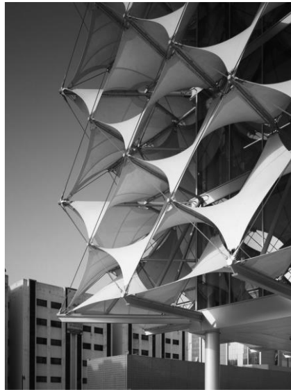
Figure 2. 5. Example of used different material on movable shading panels (Source:Srisuwan,2017)
