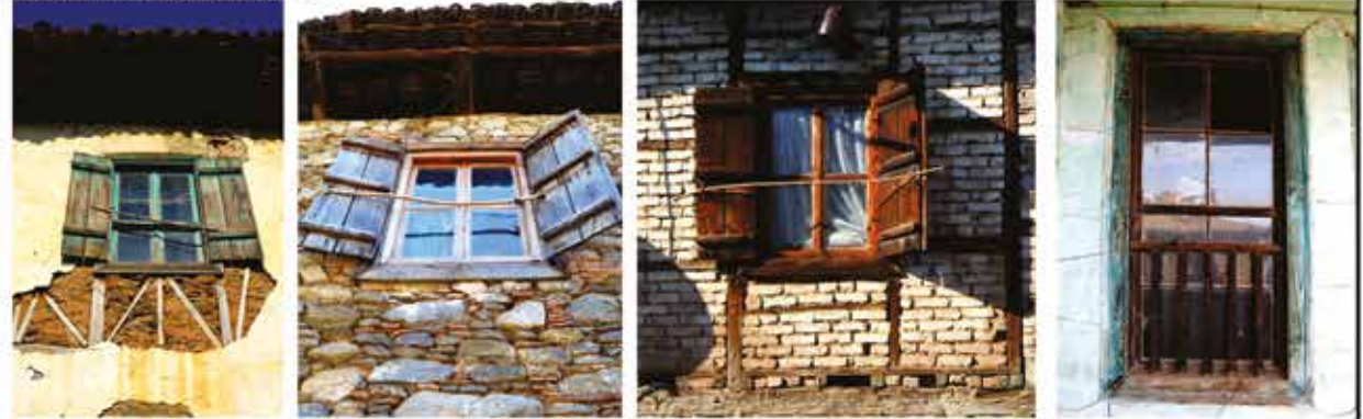
Foto. 8-15: Pencere ve kepenkler Photo. 8-15: Windows and shutters
