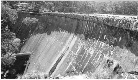
**Fig. 2.** January 30, 2000, photograph of the Lower Stony Creek Dam in Geelong, Australia (masonry dam completed in 1873):  $H = 18.3$  m,  $L = 68$  m. The dam was the first curved gravity dam in Australia. Note the low-flow spillway section in the middle of the dam crest.
